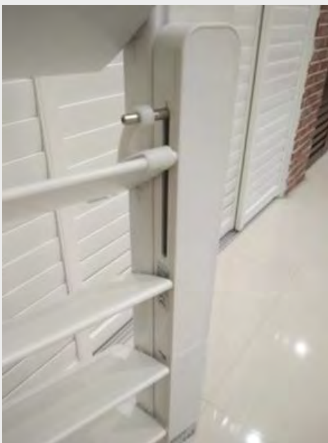
Motor Installed On Stile
