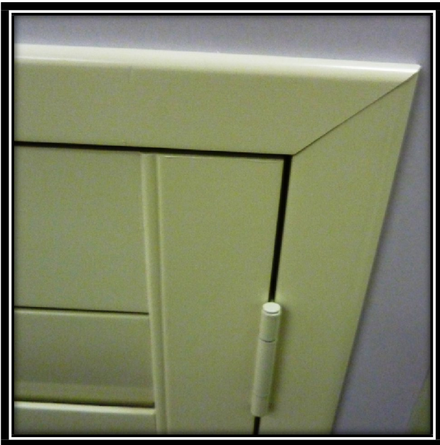
Z Sill Frame at bottom of Bullnose Z Frame
